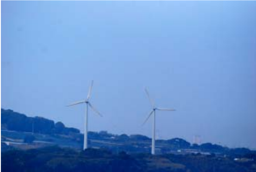
Wind power generation of Kanagawa Prefecture Miura City Miyakawa park
